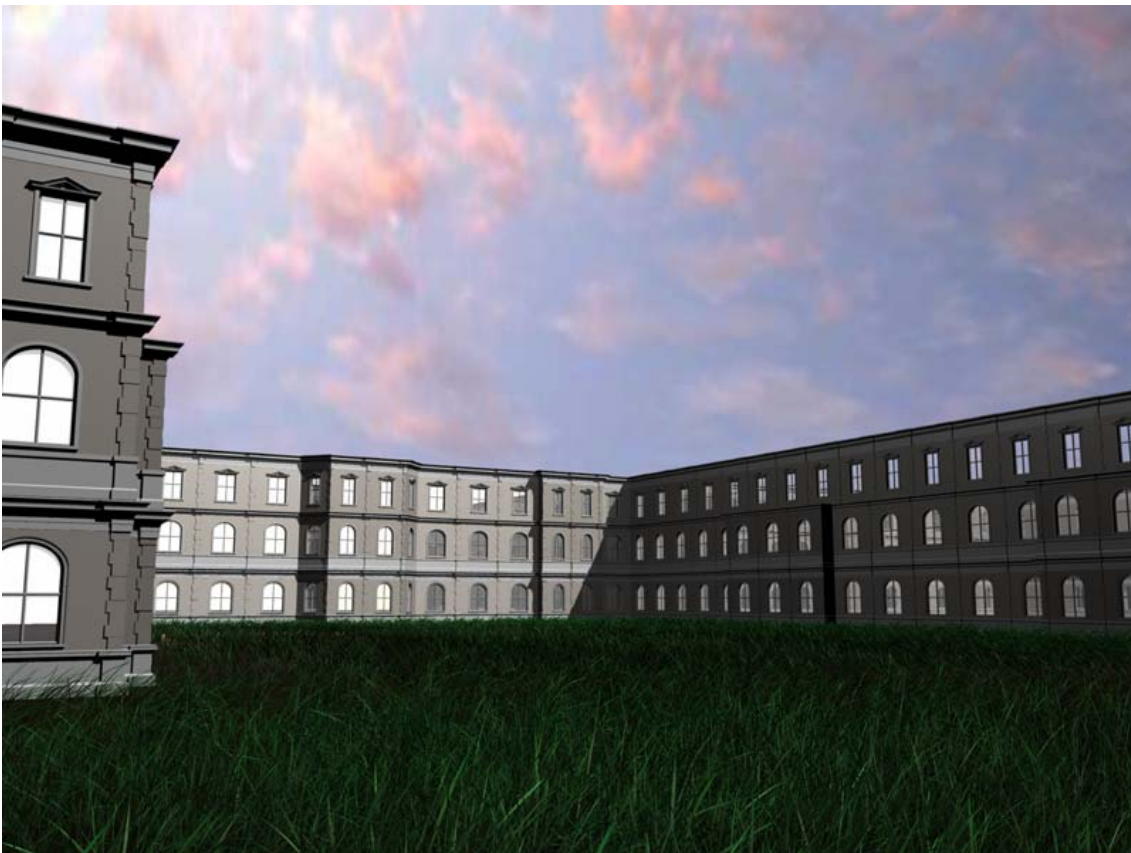
Figure 14: Example façade of a large building.
